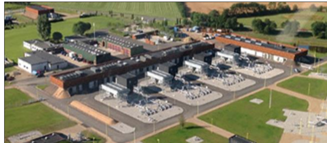
Egtved compressor station, example
