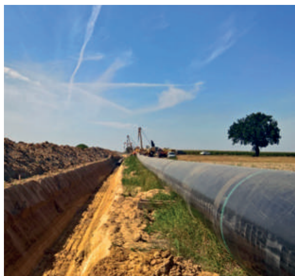
Pipe laying landscape Karolina Talaśka, Poznań Branch
