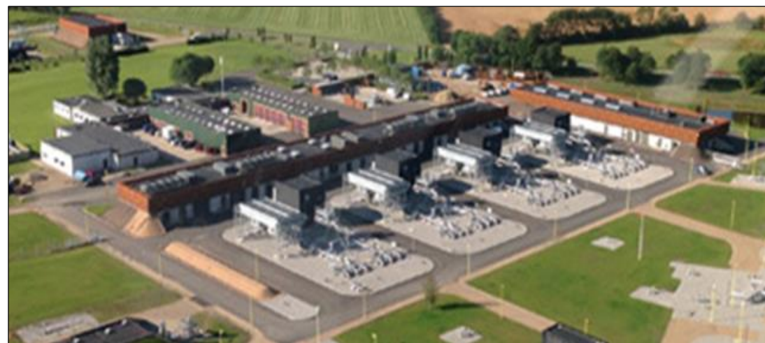
Egtved compressor station, example
